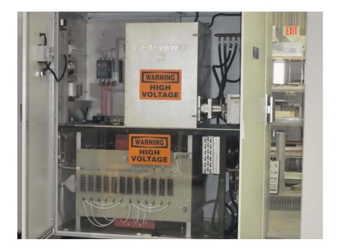
Here is the view inside of one of the transmitters. A magnetron is used to generate the RF energy. The magnetron is located in the upper center of the photo in a metal case. The RF output is on the right side of the unit, which is a waveguide flange.
